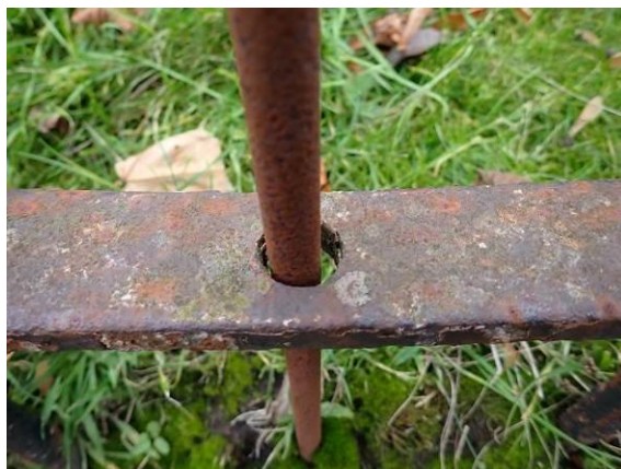
Unpassender Reparaturstab
